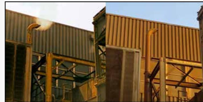
Before/after comparison: Oil mist on a gas turbine before and after the installation of an Oil Mist Separator from FRANKE-Filter.
